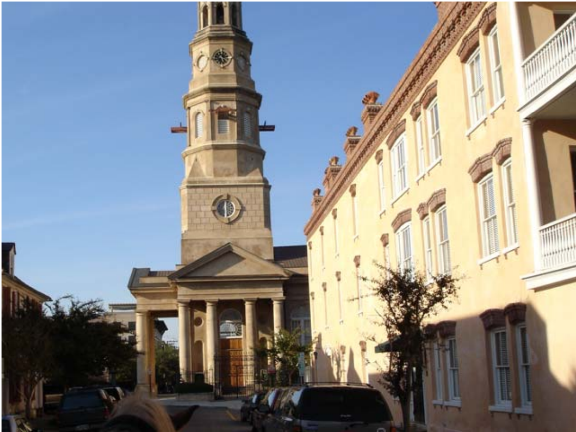
Church with supporting rods to keep it from tumbling down
